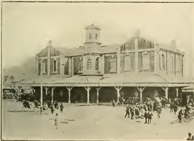
RAILWAY STATION IN JAPAN.
